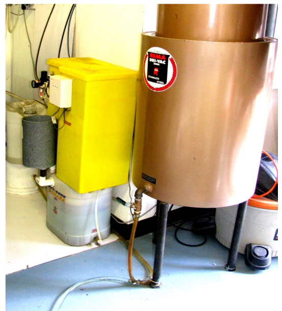
WATER INLET MANIFOLD CONNECTION TO AIR VACUUM
