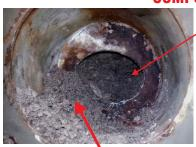
LOAD OF SCALE AT THE OPEN HAND HOLE ON A TUBELESS BOILER
